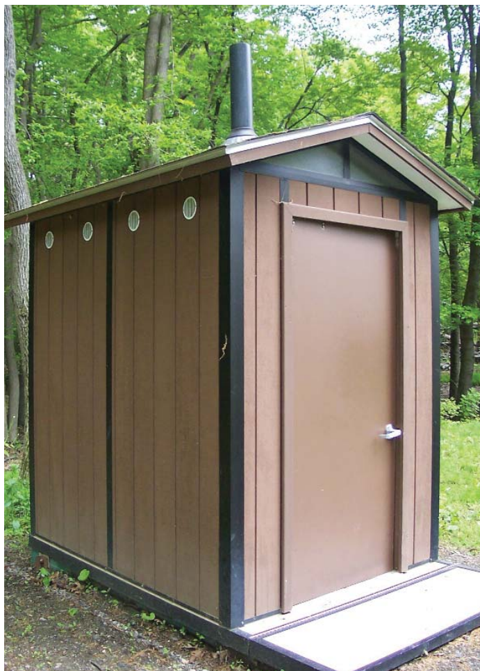
Smaller composting units can be ideal for trailhead installations.
